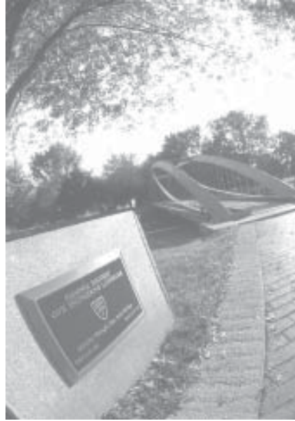
Moseley Wrought Iron Bow Truss Arch Bridge
