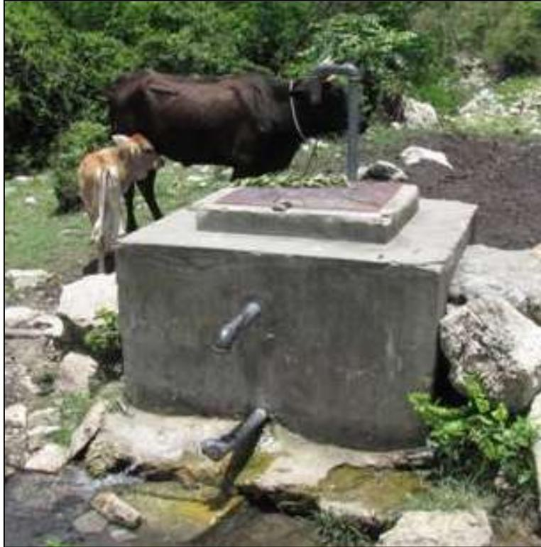
**Figure 3: Small concrete storage tanks with faucet**
